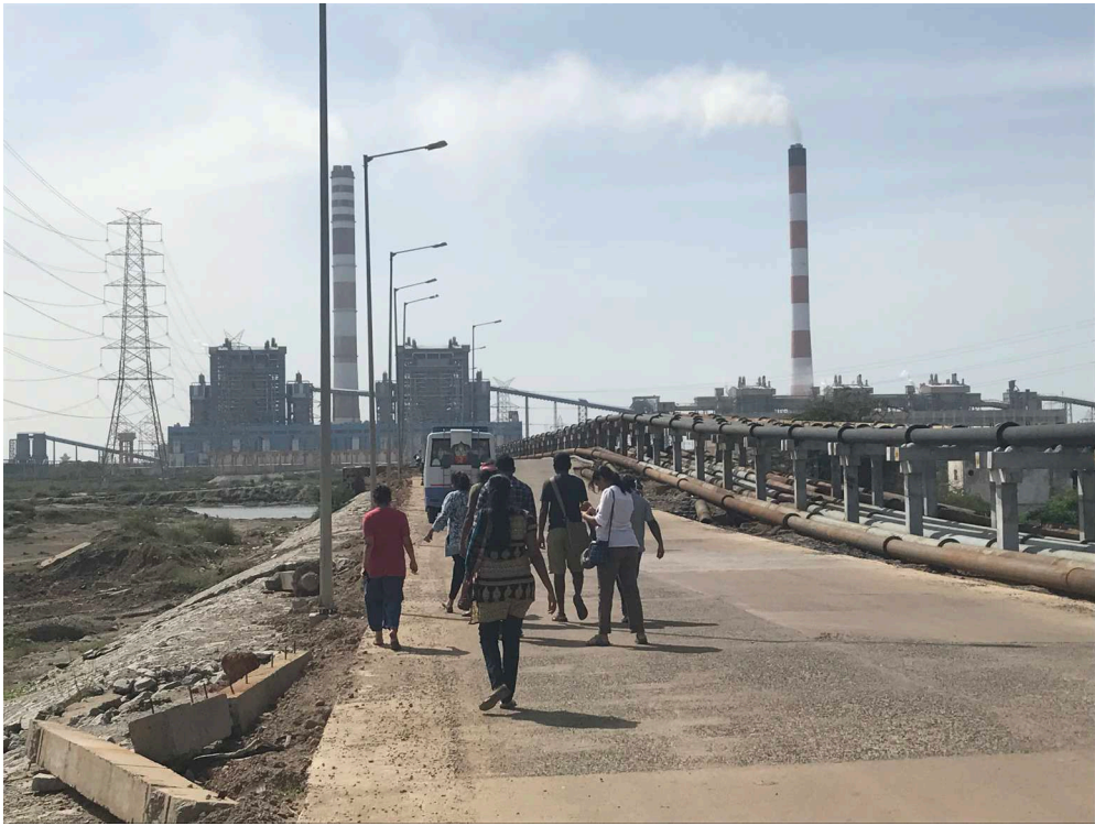
Figure 5. Ash pipeline Road, Ennore, 22 July 2017. Photograph by the author.
