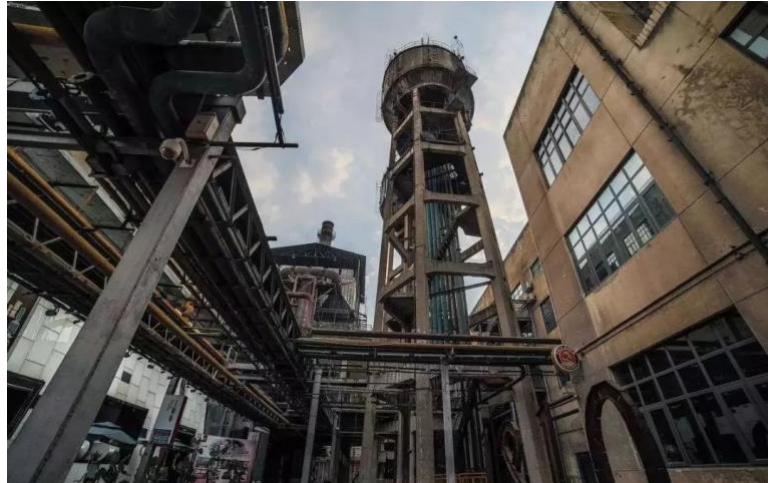
Figure 4.5 Industrial Structures of Former Hongguang Electronics Factory.
