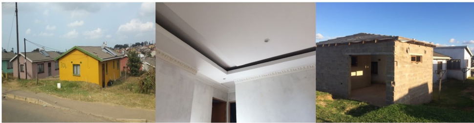
Figure 6. FEDUP households; the interior improvements and extensions in Namibia Stop 8.
