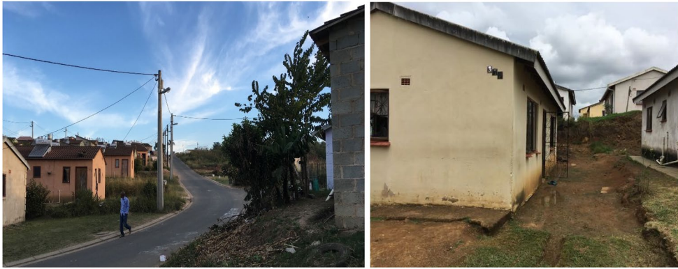
Figure 2. Namibia Stop 8 (Inanda, Durban Metropolitan Area).
