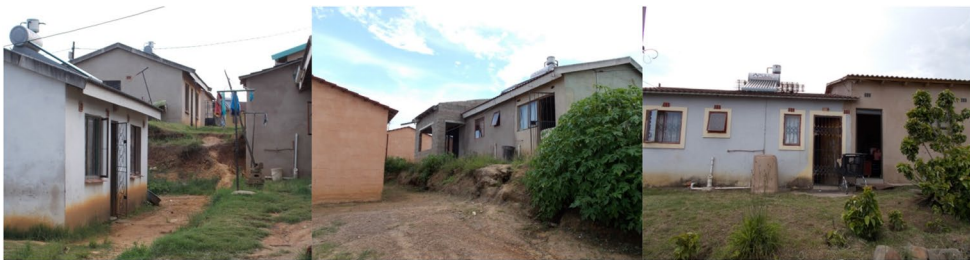
Figure 7. Views of the passages showing their poor condition, lack of boundaries and the encroachment into people's yards.
