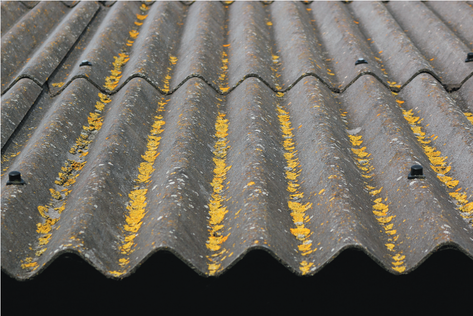
FIGURE 2 The micro garden on the roof of Lichen House, an early soil.
