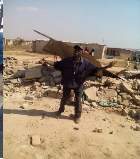
Epworth houses bulldozed
