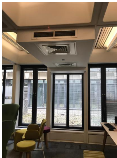
Fig. 6 – Cooling units installed between coffered ceiling panels
