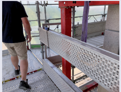
Well-protected scaffolding platform on Copenhagen refurbishment site
