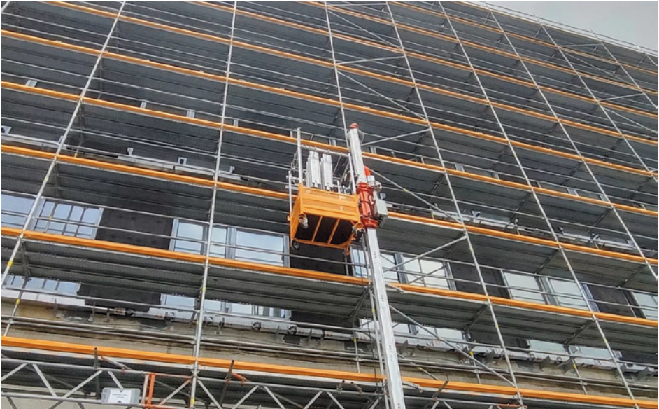
New technologies: Alimak's scaffolding transportation system Courtesy of VSB
