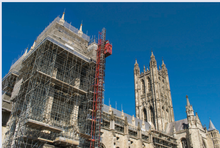
Scaffolding on Canterbury Cathedral, England, dating back to 11 th century
