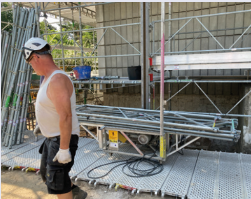
Scaffolding with hoist on Copenhagen refurbishment site
