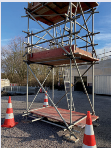
Tube and fittings: the mother of all scaffolds
