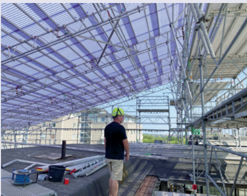
Complex scaffolding on roof of Copenhagen refurbishment site
