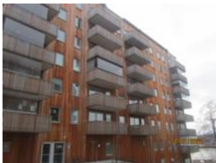
Photo 6: ARVET wood construction project in Stockholm
