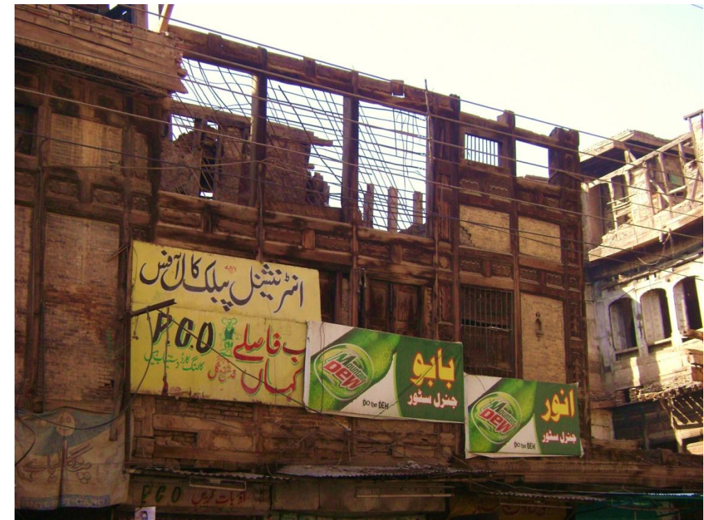
Fig. 6.11 Depleted haveli showing structural members on Bazaar-e-Kalan road, Peshawar.
