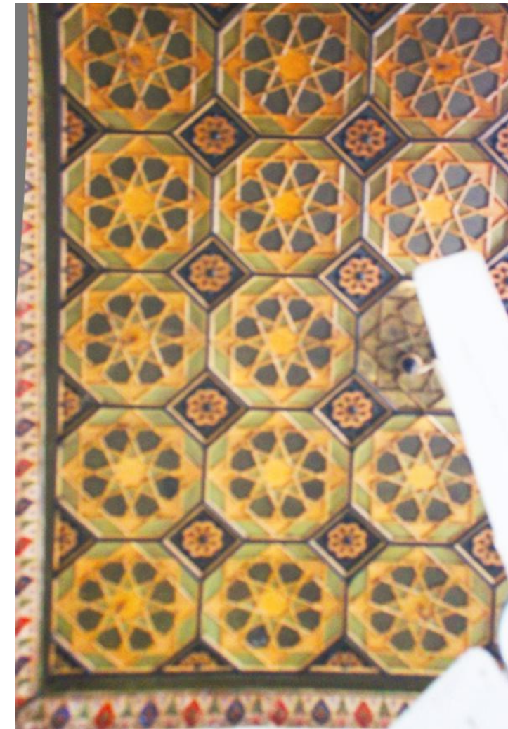
Fig. 8.121 Khatam-band ceiling of south dalan .
