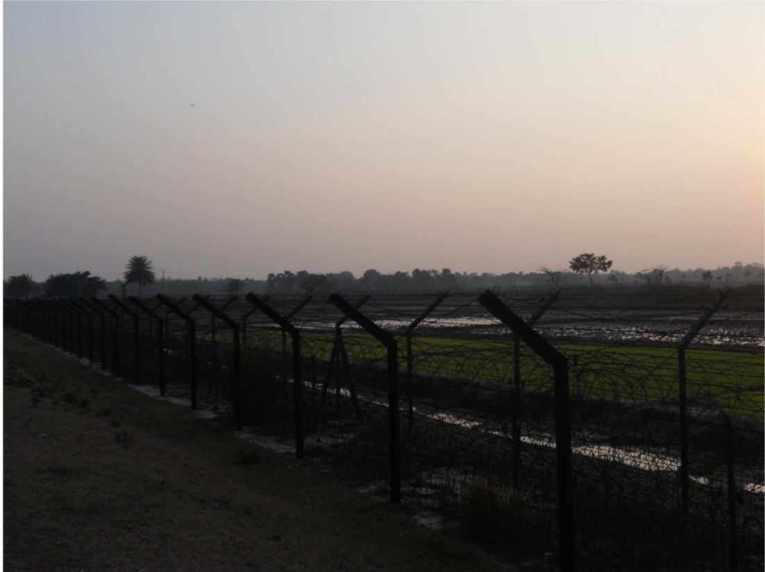
Plate 5. Fencing along the South Dinajpur border, West Bengal, 2012.
