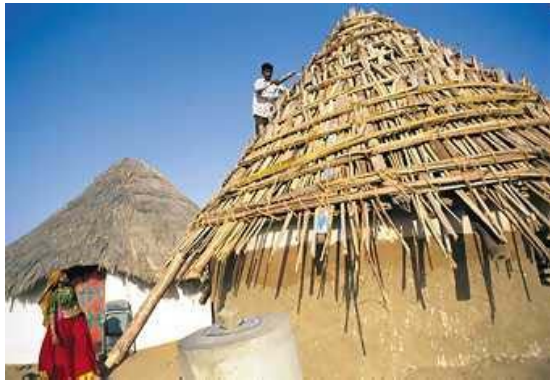
Figure 2.8 People in Kutch constructing their houses (bhoongas) using mud material.
