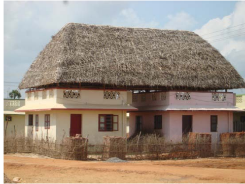
Figure 6.35 A and B In order to accommodate joint family of 11 members, people extended their house on first floor with thatched roof.
