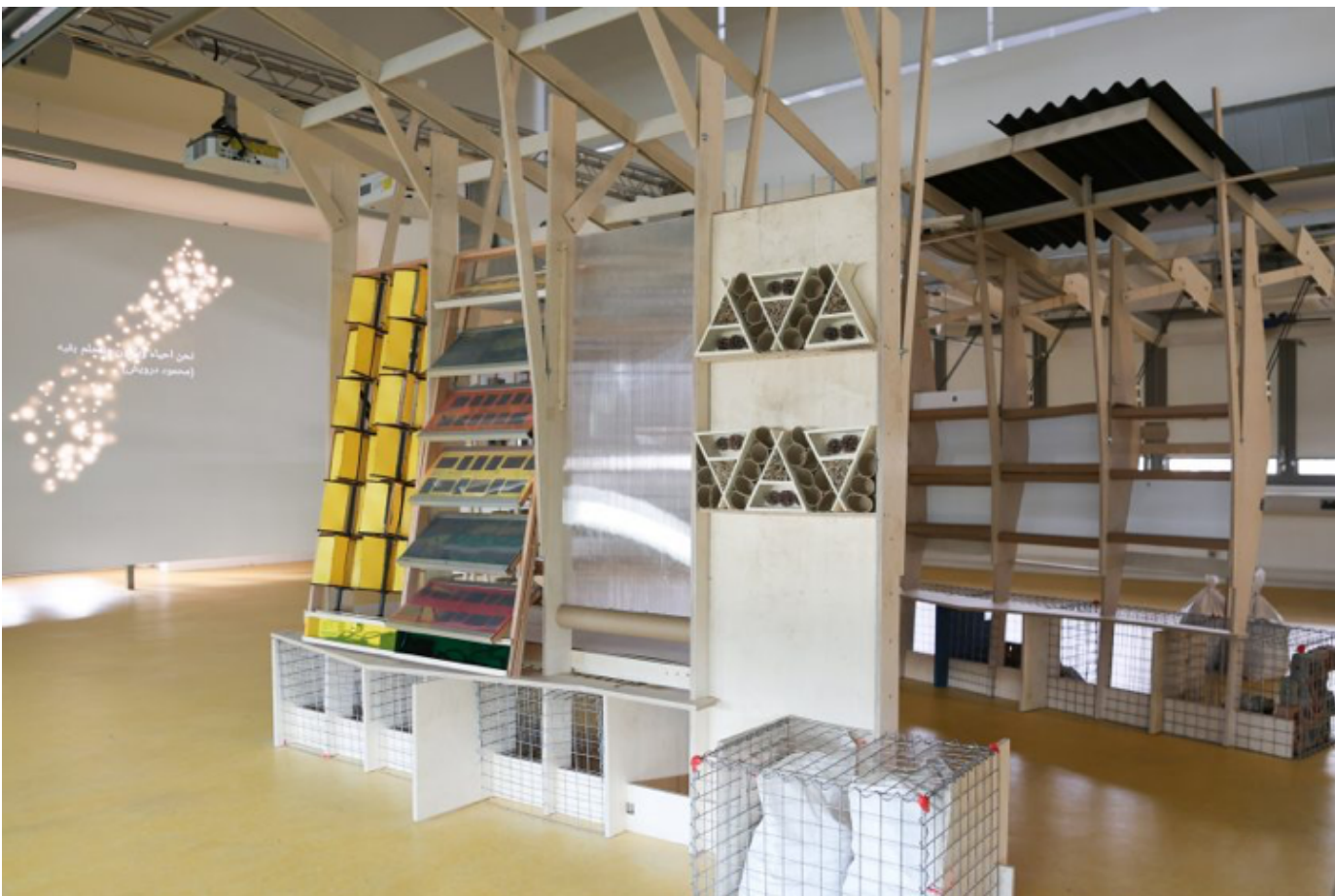
Rubble-filled gabion baskets form the foundations
