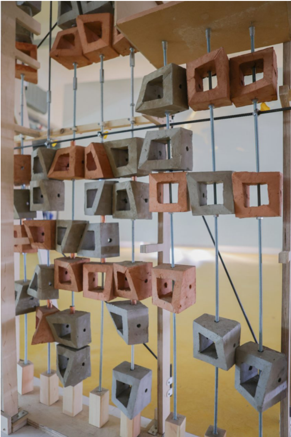
Clay modules fitted around water pipes provide evaporative cooling
