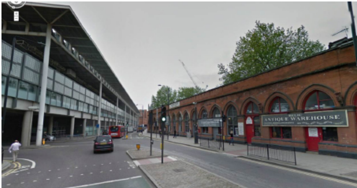
Fig. 7.2. St Pancras International Station, left, and 119-149 Pancras Way shops, right
