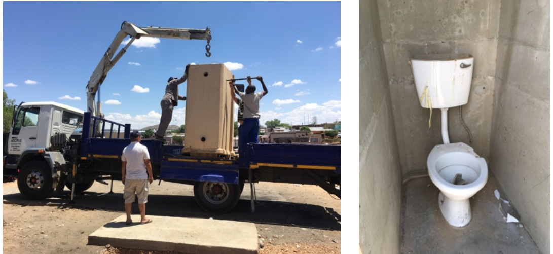
Figure 33: Installation of the toilets by the external contractor (left) and interior of newly installed cubicle with broken fittings (right).
