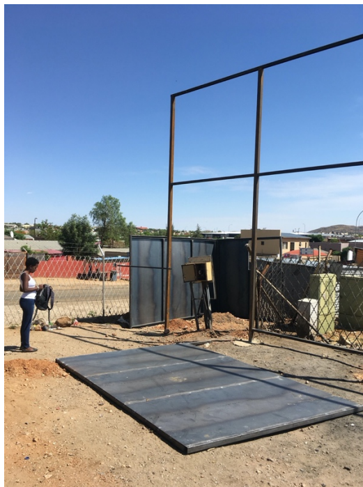
Figure 52: Prefabricated wall panels of the office during assembly with billboard frame already in place (left), and construction of the frame of the meeting hall (right).
