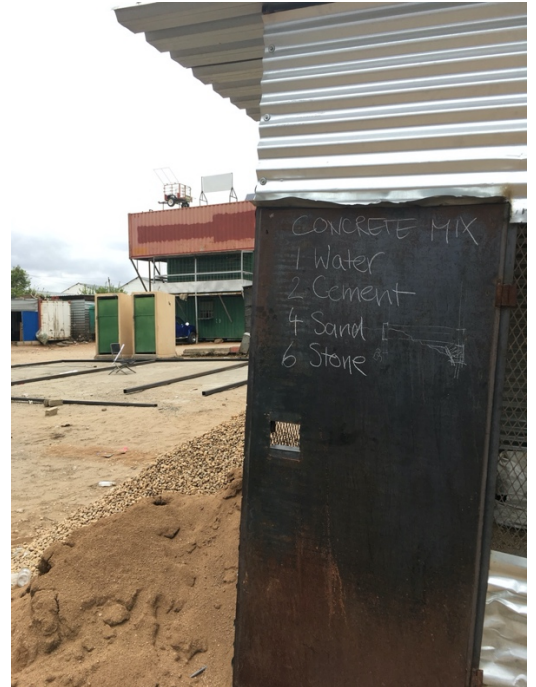
Figure 51: Prefabrication of the billboard steel frame on the concrete surface of the disused car wash (left). The concrete mix recipe written with chalk on the door of the neighbouring building (right).
