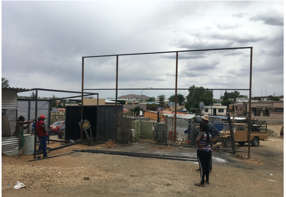
Figure 53: The frame of the meeting hall partly clad on the street facade.
