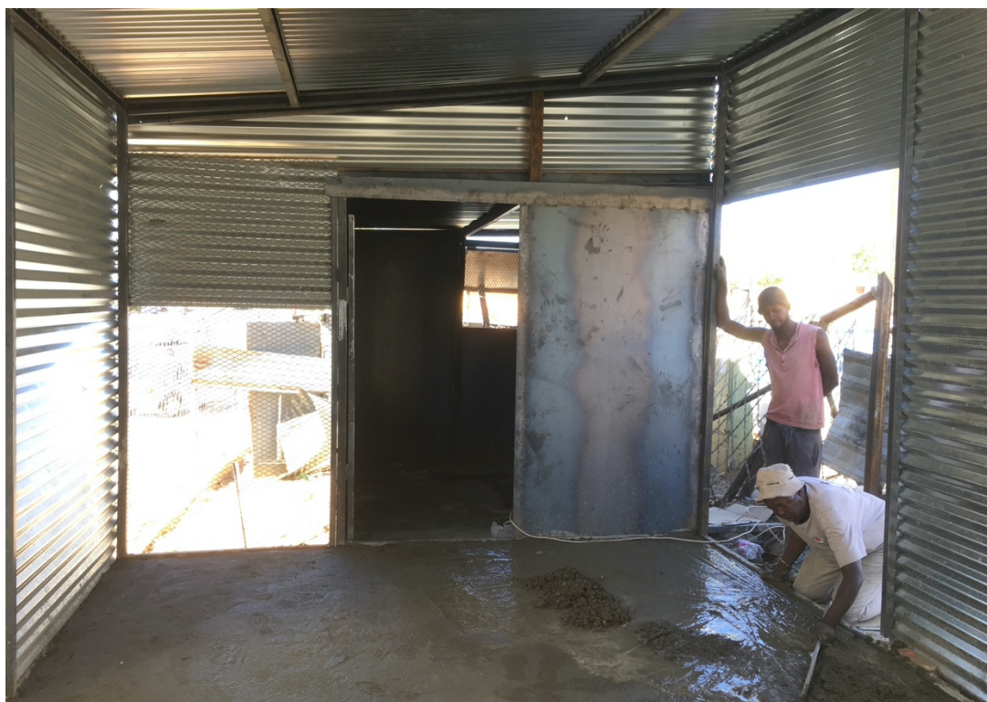
Figure 56: The concrete floor of the meeting hall being cast and finished.
