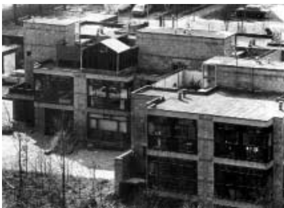
8 Genter Strasse, Munich (1972) by Otto Steidle with Doris and Ralph Thut; frame and infill
