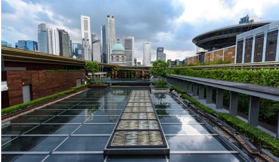
Figure 7. The new roofscape with a view towards the dome of the former Supreme Court in the distance and the disk-like roof form of the current Supreme Court on the right.
