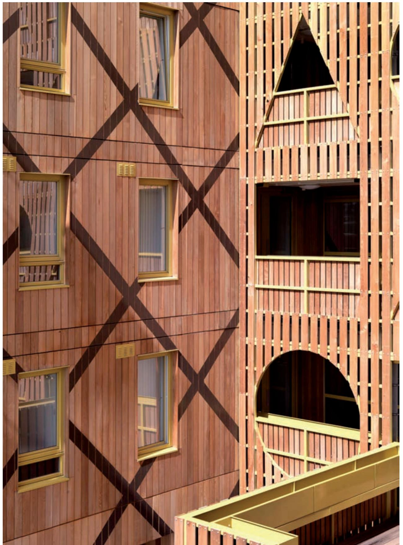
Fig. 38 Timber cladding detail 1, photograph Charles Hosea
