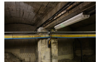
Figure 11. York Street vaults, Roman baths: a meeting place of spatial intervention across millennia.
