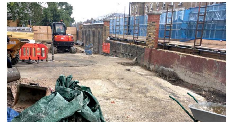
Fig. 32 Eleanor Palmer Science Lab, at the start of the build showing scaffold supporting the boundary wall from collapse
