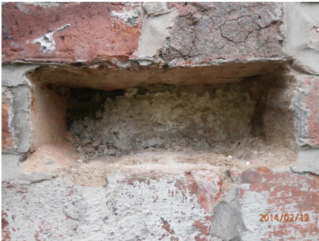
Figure 4: Opening revealed following removal of brick. The amount of mortar present, the presence and position of any frogs and other internal features were examined.
