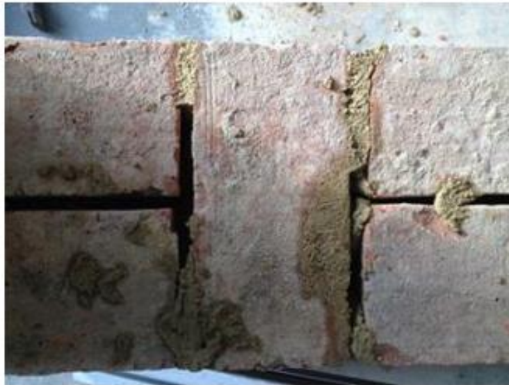
Figure 9: Partially filled joints were deliberately included in some of the test walls which were built for testing in the NPL hot-box apparatus.
