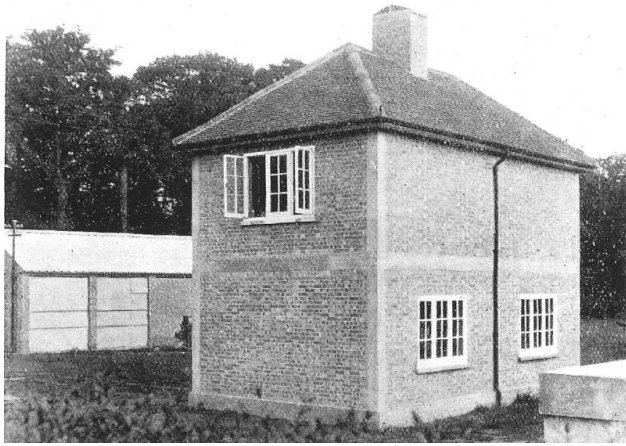
Figure 3: The BRS experimental house (left), informally known as ‘Fishenden House’, and the BRS wall laboratory (right) used to provide initial data which formed the first established U-value coefficients. Initial results were provided from the experimental house, with the wall laboratory established to undertake more comprehensive experiments (from Dufton, 1933 and Dufton, 1941). More detailed description of the wall laboratory can be found in Pratt, 1981.
