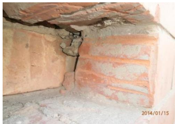
Figures 16 and 17: The use of broken bricks / brick bats on the inner leaf ( left ) and in place of a full header brick ( right ) introduce air cavities into the wall structure. These types of features were found in ~9% of walls examined.
