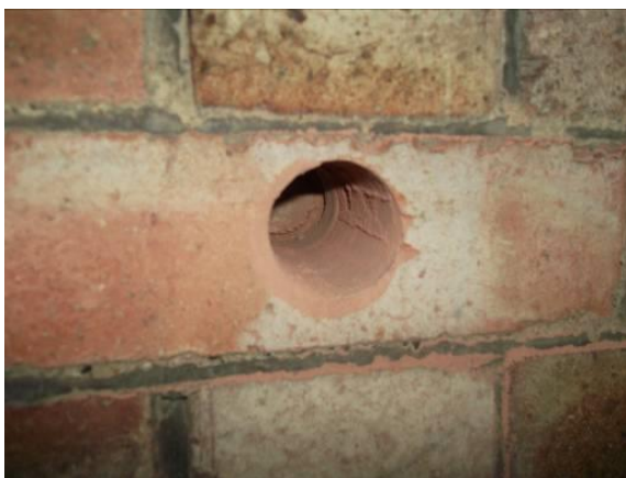
Figure 5: An area where a core sample was taken. The gap between the inner and outer stretchers is just discernible as a shadow at the back of the bore hole.
