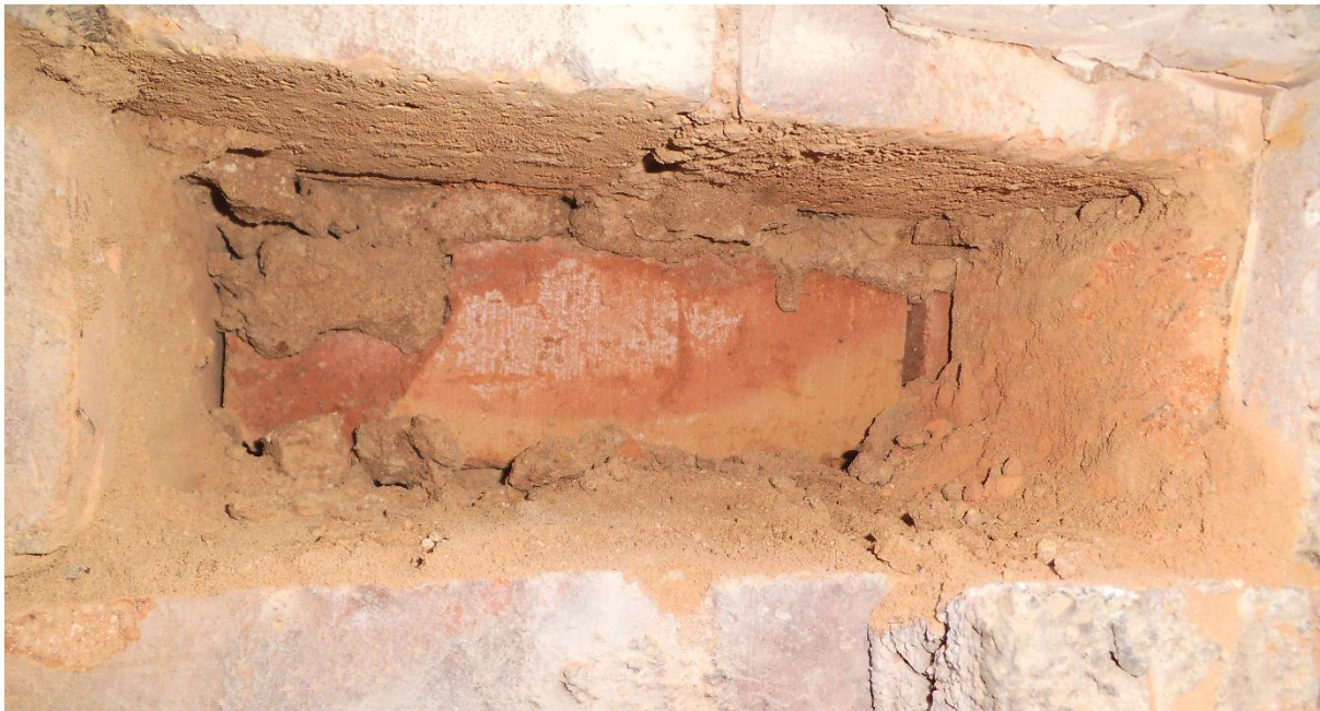
Figure 8: Exposed collar joint showing area of missing mortar. Some mortar remains attached (e.g. in the top left of the exposed inner leaf), with other regions showing staining (e.g. bottom right of the exposed inner leaf). The central portion of the inner leaf shows no staining, suggesting little or no mortar was present.
