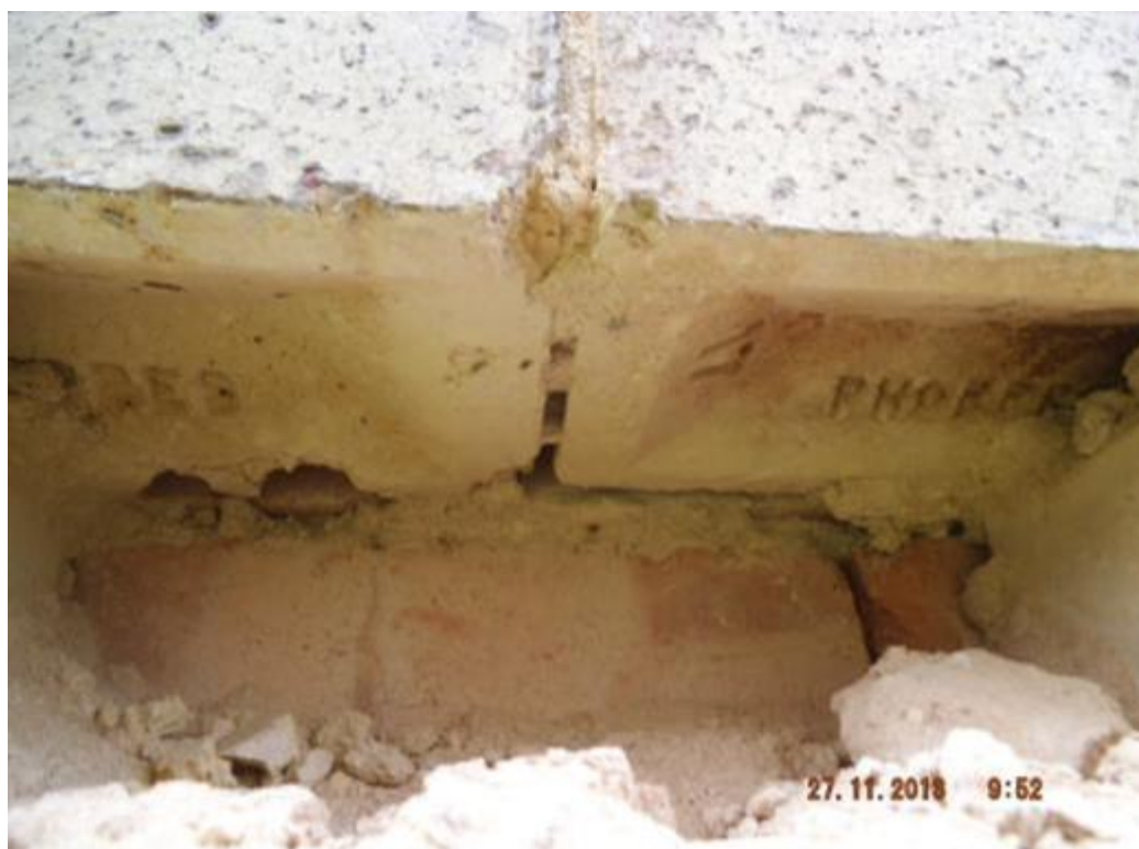
Figure 12: Frog-down bricks. The cavity created by the frog in the brick is clearly visible. The on-site technicians were able to ascertain that any cavity was genuine (and not simply created by falling mortar following the brick removal) by looking along the course. This example also shows evidence of an imperfect brick being used (the back face of the upper left brick in the in the upper course is broken) – see below.
