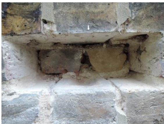
Figures 16 and 17: The use of broken bricks / brick bats on the inner leaf ( left ) and in place of a full header brick ( right ) introduce air cavities into the wall structure. These types of features were found in ~9% of walls examined.
