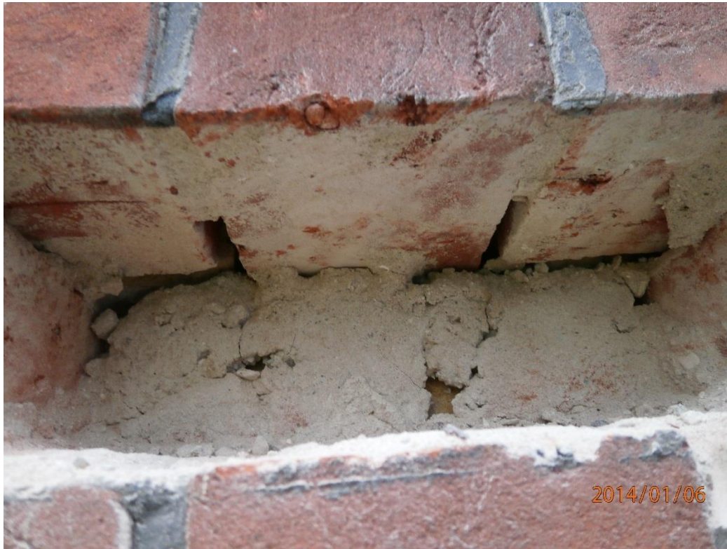
Figure 10: Example of missing mortar in perpend joints. Looking upwards at exposed bricks in the upper course at the top of the void, the extent of mortar in the perpend joints can be seen. In this example, the perpends can be estimated to be approximately 50% filled.
