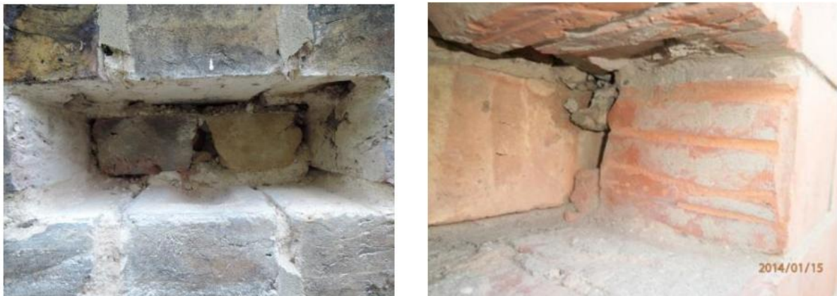
Figure 5: Examples of air gaps within the walls visited as part of the Report 2 fieldwork, created by the use of broken bricks ('brick bats'). A single lengthways 'stretcher' brick was removed from the wall and the internal condition of the wall was examined. On the left the use of broken bricks in the inner leaf can be seen clearly. The photograph on the right shows the use of a 'snapped header' - i.e. one which appears to be a header (end on) brick but which in fact has been snapped and is only half the original length, generating an additional joint and air gap.
