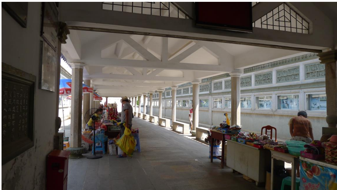
Figure 1: The roofed corridor with stone carvings displayed on its both sides (photo by author)
