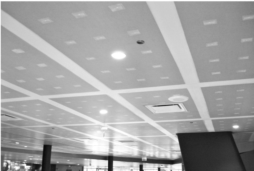
fig. 18. McCormick Tribune Campus Center , Campus of the Illinois Institute of Technology, Chicago: Office for Metropolitan Architecture, 2003; unpainted sheetrock panels
