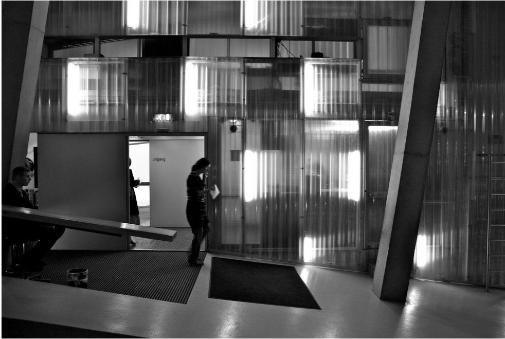
fig. 17. Kunsthal , Rotterdam, Netherlands: Office for Metropolitan Architecture, 1992: corrugated polycarbonate panels
