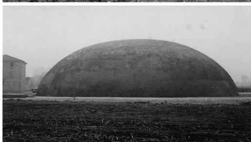
Figure 8. Pictures showing the ‘inflation’ of the first 30 m diameter Binishell dome by Dante Bini. Castelfranco Emilia, Italy, 1968. Dante Bini Archive.
