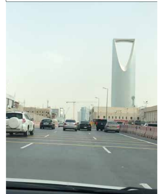
Figure 87.b: The Kingdom Tower as it appears from Olaya Street; direction towards S. (source: Author).
