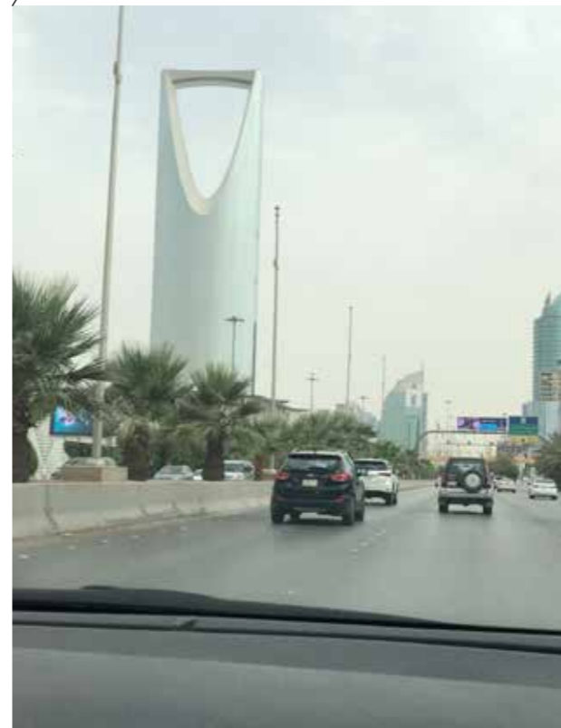
Figure 87.a: The Kingdom Tower as it appears from King Fahad Road; direction towards S. (source: Author).
