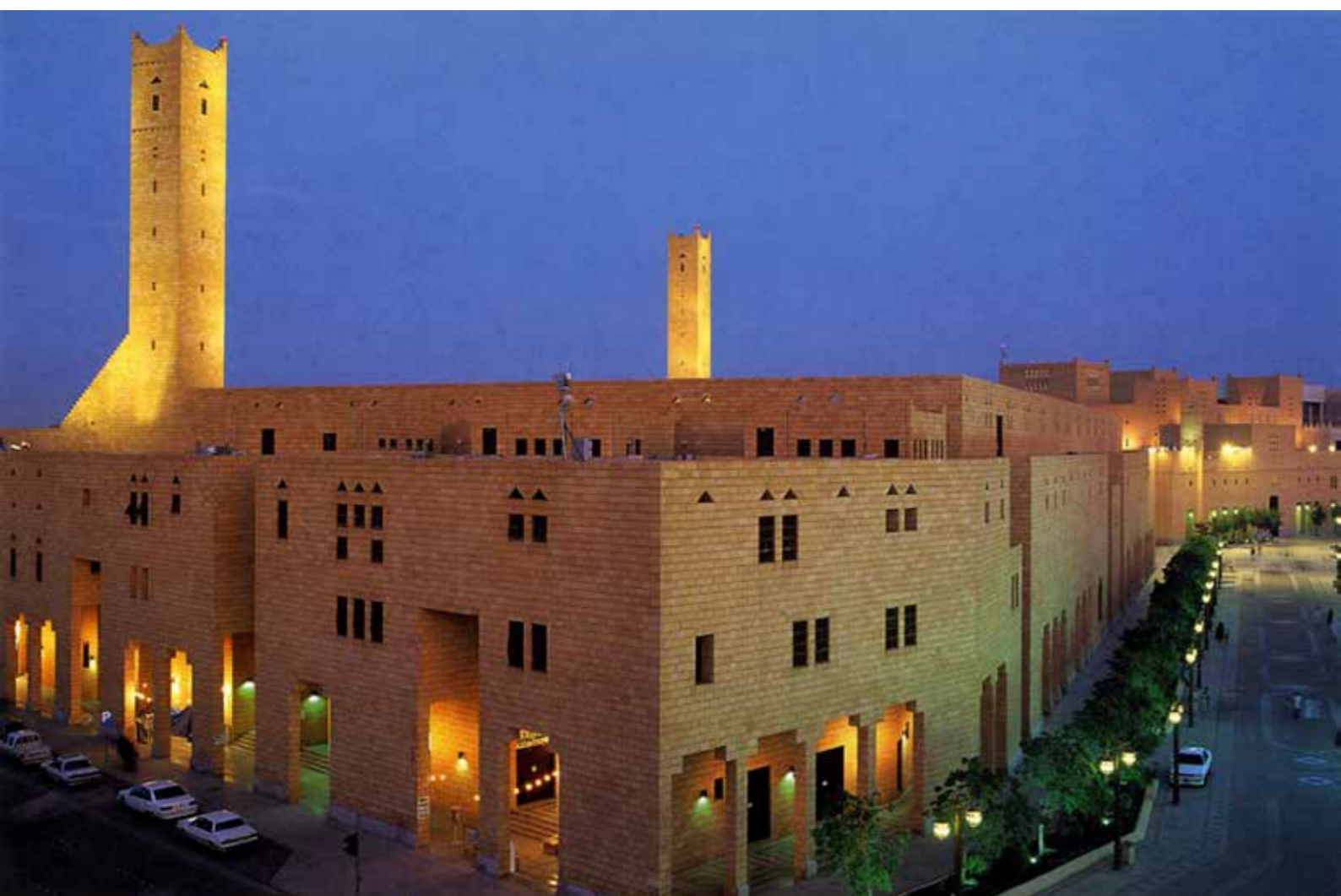
Figure 31: Redeveloped Grand Mosque in the old centre of Riyadh (source: Badran, 1992)..
