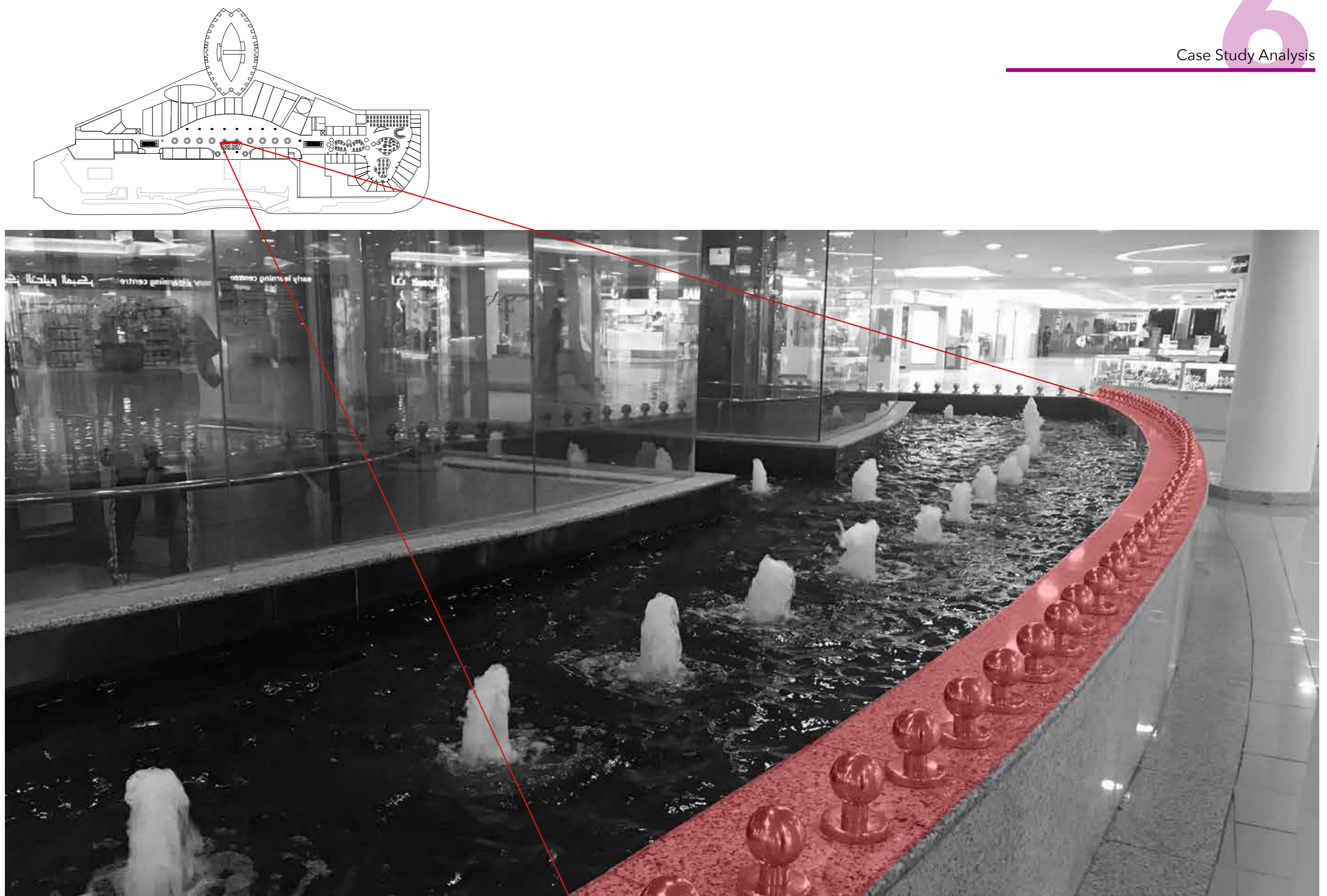
Figure 100: Decorative elements are meant to prevent customers from utilising the edges as resting benches (source: Author).
