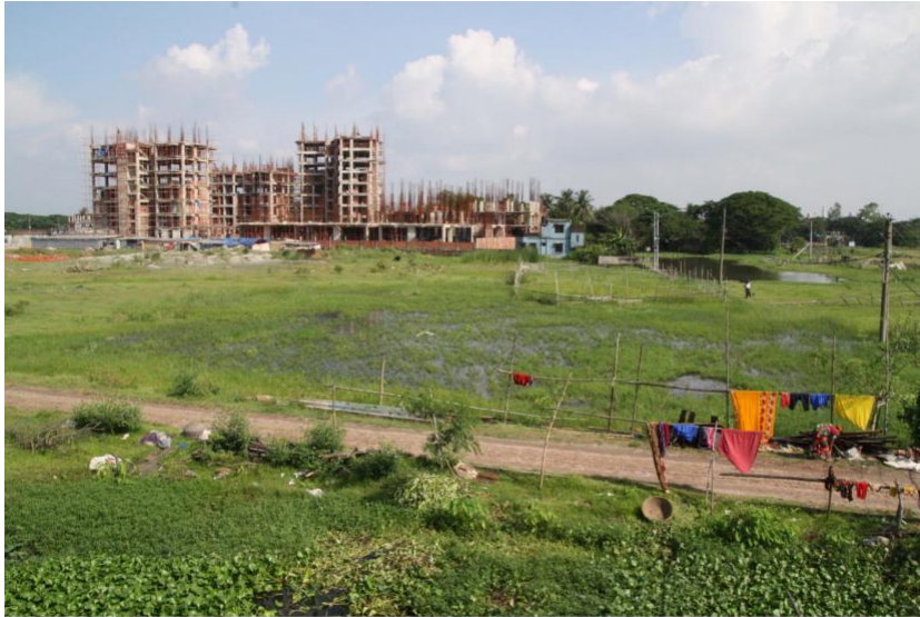
Construction on wetlands, Madani Avenue. Photo: Beth Cullen.
