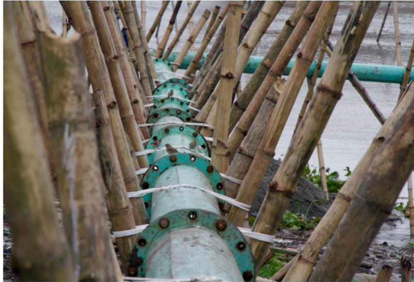
Sand pipe, Turag River. Photo: Beth Cullen.
