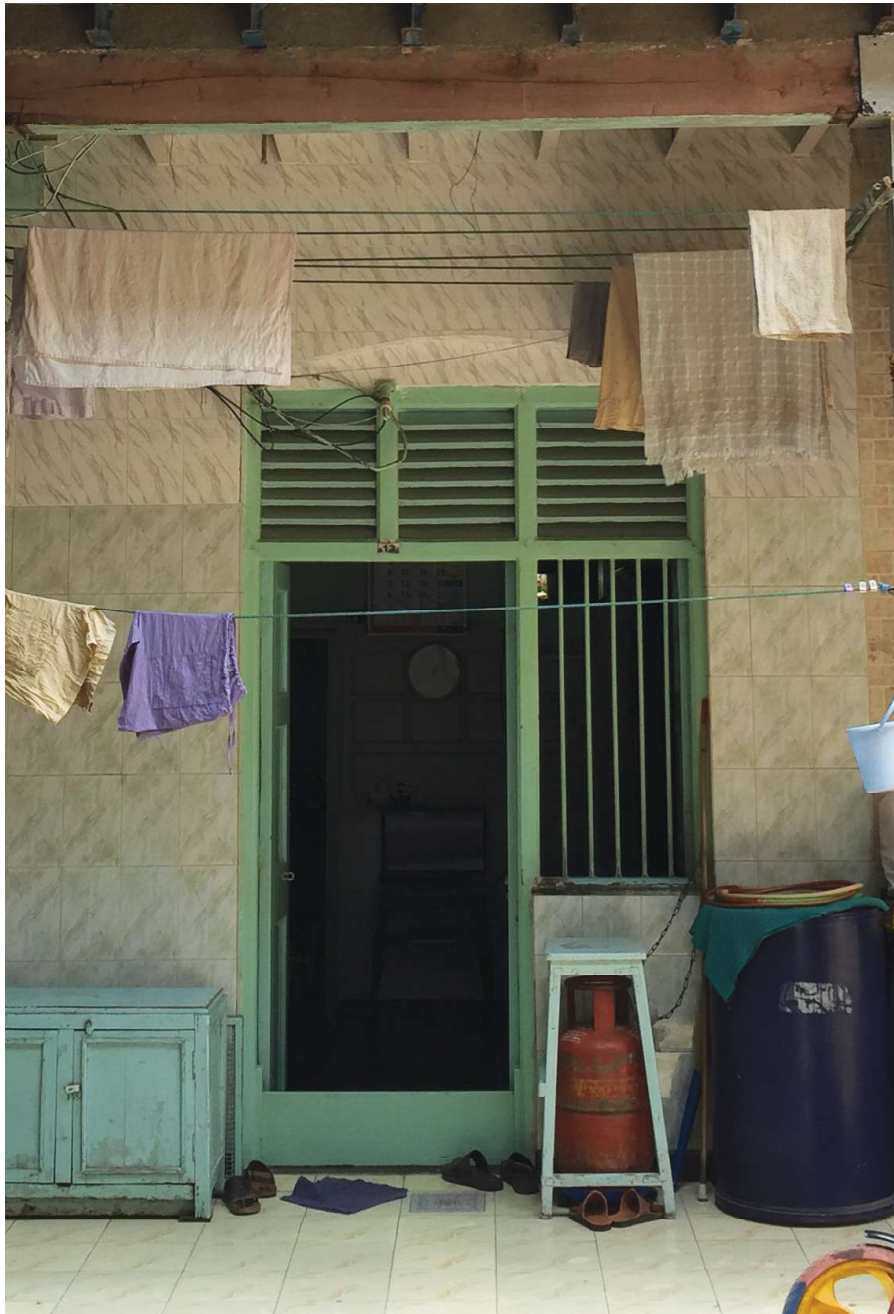
Fig.5.58. The Door + Window + Ventilator Combo
