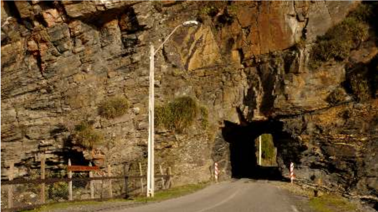
Figure 3.15: Sacred place of the Pucatruhuequeches and the tunnel of Pucatrihue. This tunnel was made using explosives constituting the origin of the San Pedro fishermen cove. Picture extracted from UHD video
