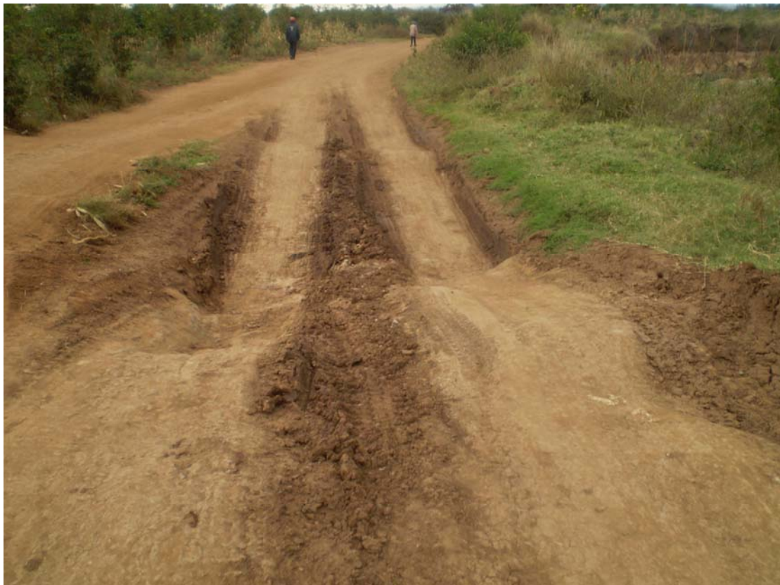
Plate 3: A section of the main access road into Miarau quarries.
