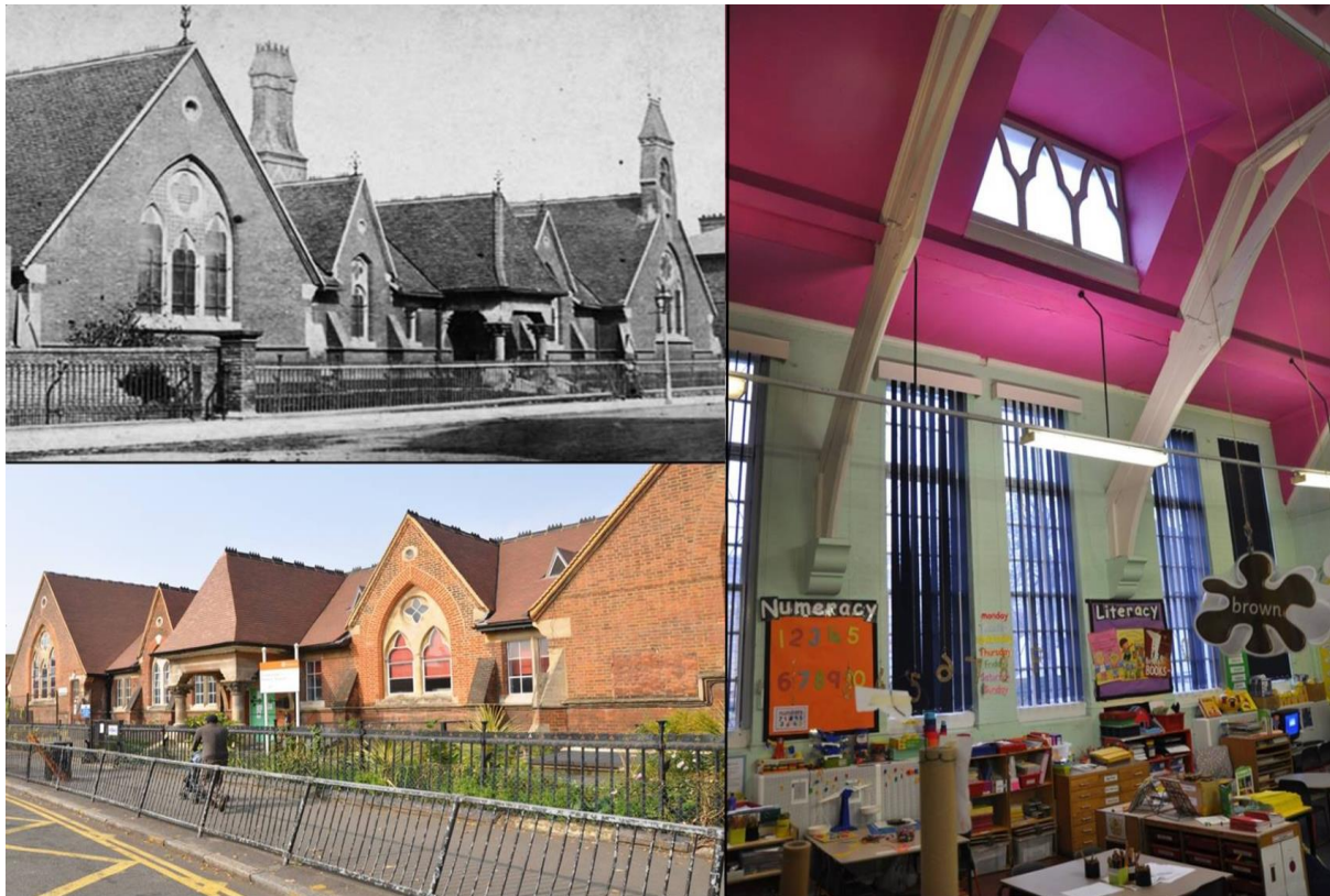
Figure 4. The 6th, Kingsland, Birkbeck School, constructed 1852. Above left: c 1880 (courtesy of Hackney Archives) and below: as Colvestone Primary School today. Except for the removal of the belltower and chimney the façade and much of the fabric is original. Right: a classroom today showing rooflight and ventilation (author’s originals).
