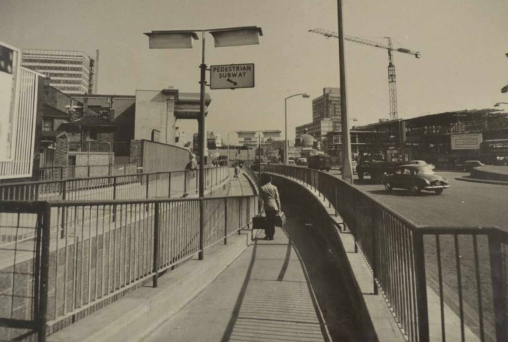
FIG.15. Image taken by Southwark Public Libraries, in Nov. 1963. Elephant and Castle redevelopment, showing progress on the new Shopping Centre. Showing the former public subways closed in 2015
