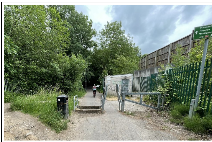
Figure 1. Access control barriers across a traffic-free walking, wheeling and cycling path in Stockport, Greater Manchester.
