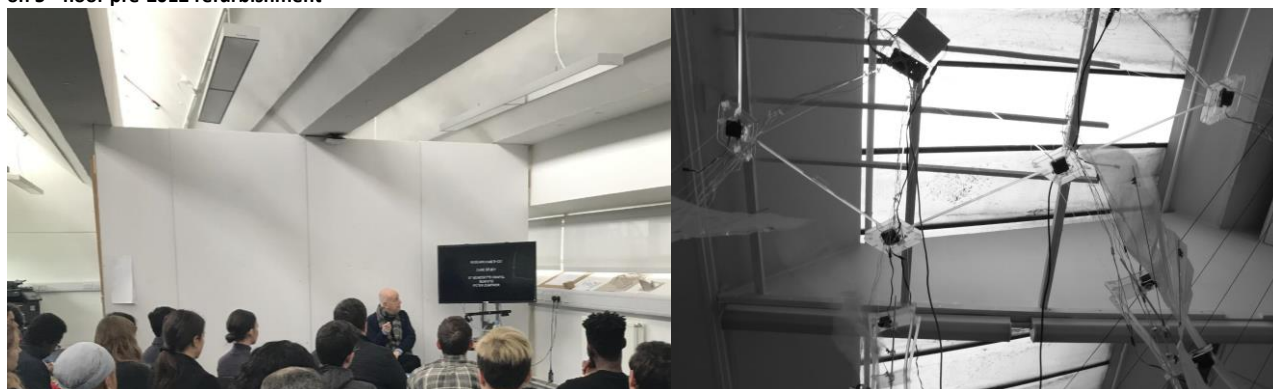
Figure 3 - (left) saw-tooth ceiling of 6 th floor studio with vertical north facing rooflights; (right) original Georgian style wired-glass fixed roof-lights on 5 th floor pre-2012 refurbishment
