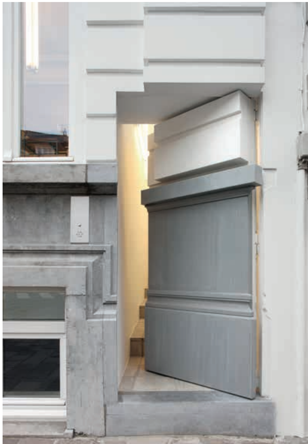
Architecten De Vylder Vinck Taillieu, Twiggy, Gent, 2012. Dettaglio della porta d'accesso al cortile | Detail of the courtyard access door. Ph. Philip Dujardin, 2012.
