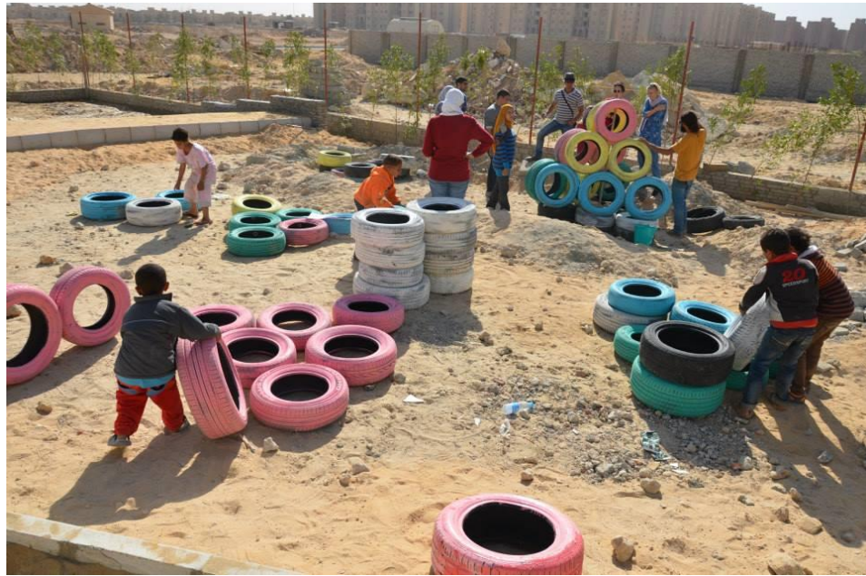
Figure 6.10 The children participating in the construction of the playing elements using recycled tyres (source: Takween ICD)
