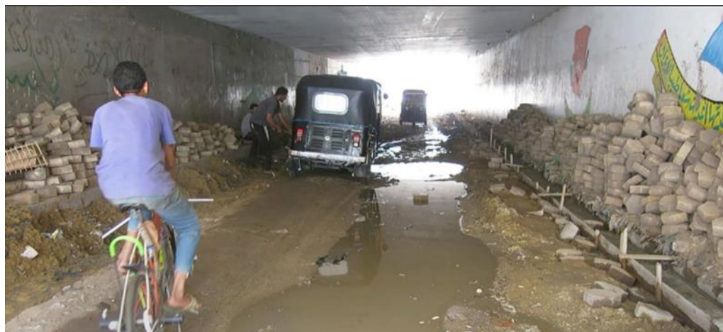
Figure 4.8 Omar Ibn ElKahtab Tunnel before intervention (source: Takween ICD)
