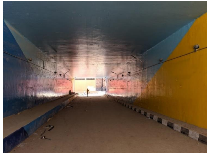
Figure 7.23 One of the other tunnels renovated by the local government (source: author)
