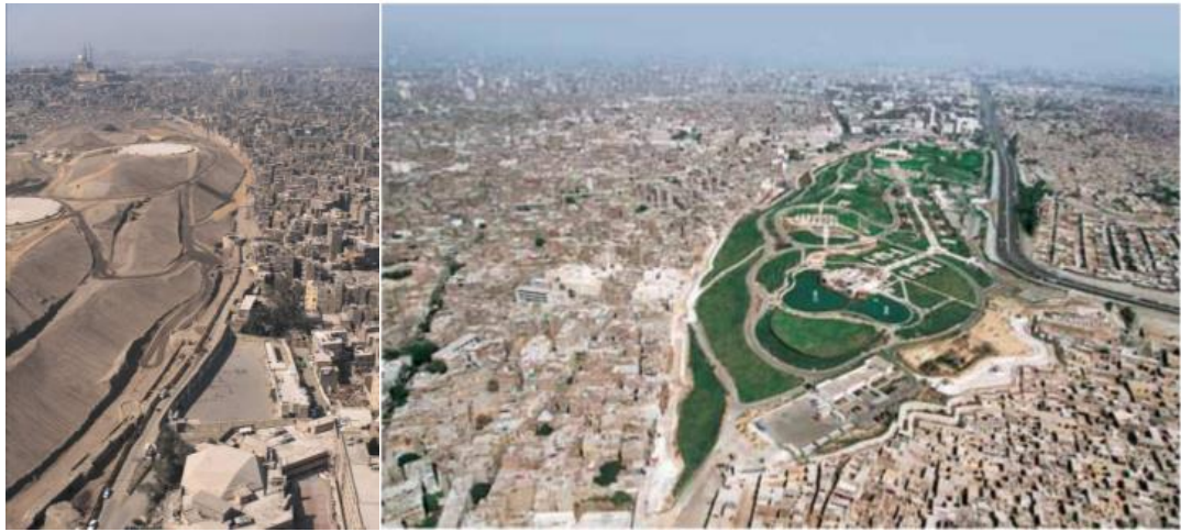
Figure 3.16 Al-Azhar park area before and after implementation (source: AKTC)
