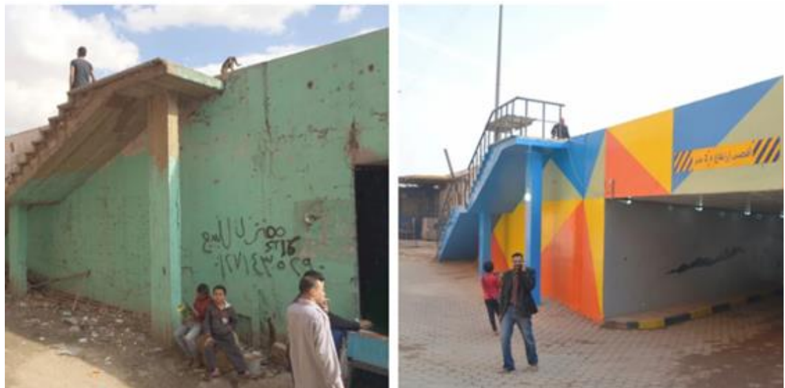
Figure 7.10 Staircase to the Ring Road before and after the intervention (source: Takween ICD)
