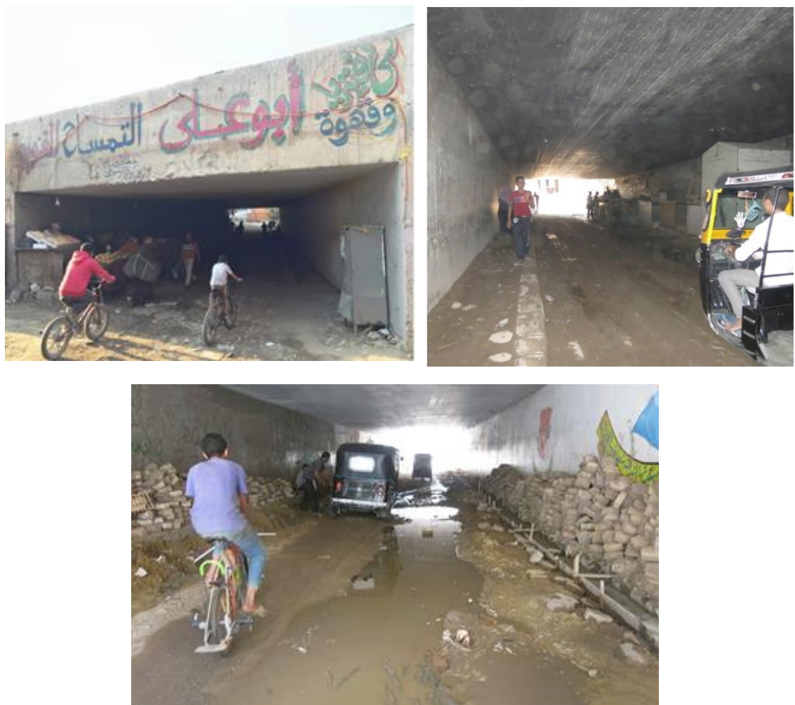
Figure 7.5 Omar Ibn Elkhatab tunnel before the intervention (source: Takween ICD)
