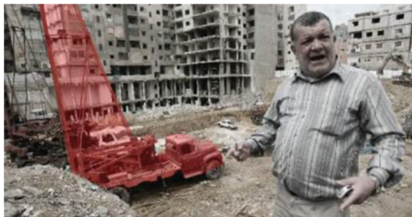
Figure 5. Site image of pile driver. image credit to al-akhbar.com.
