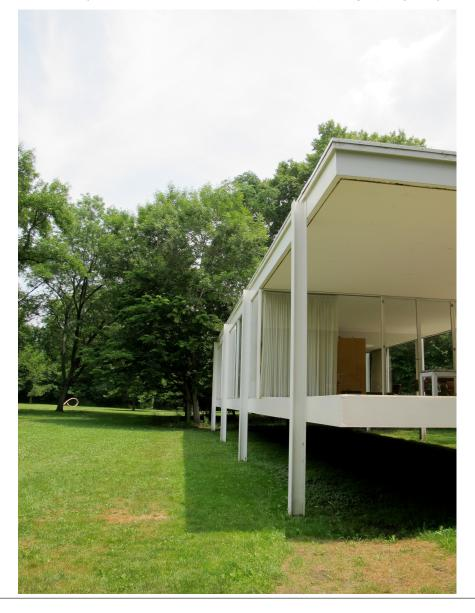
Figure 3. Column/beam junction, Farnsworth House (Source: photograph by Benjamin Lipsman)<sup>28</sup>
