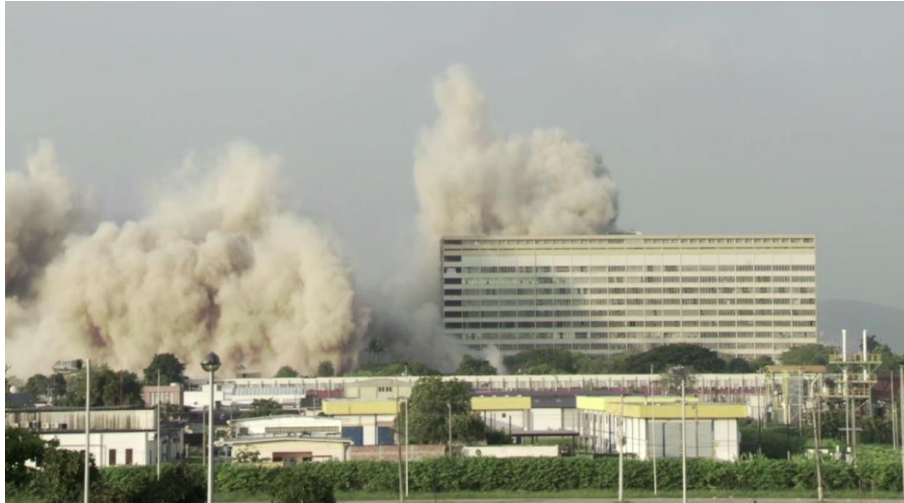
Figures 72 and 73 – The final collapse of the lame-lag
