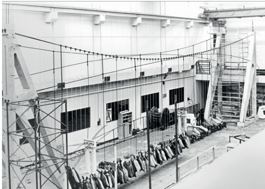
Testing concrete at Ambika P3, 1972
