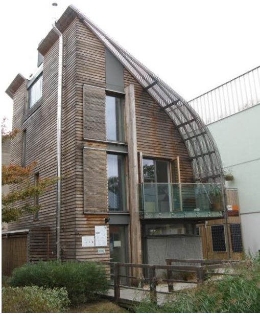
Photo: BRE Innovation Park
