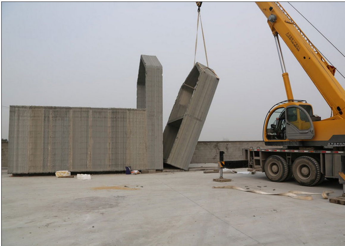
Figure 11: Yingchuang New Materials research. 3D-printed buildings using recycled materials. Image source: Yingchuang New Materials. Image source: http://static.dezeen.com/uploads/2014/04/3D-printed-buildings-China_dezeen_ss_6.jpg .
