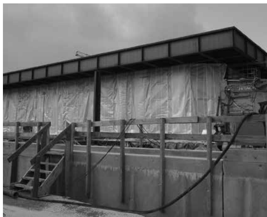
Fig.2 View of the NNG in the course of the restoration process, with polythene sheets hanging down from the roof-grid in place of the curtain-wall system
