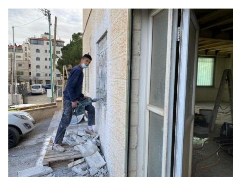
**Photo 8. 6:** A worker uses a Kangoo electric drill to open a window in a constructed wall without wearing appropriate personal protective equipment
