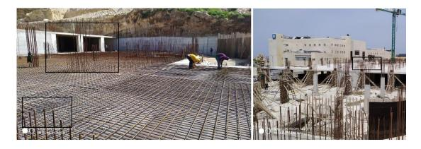
**Photo 9. 7:** Non-use of approved rebar safety caps during construction
