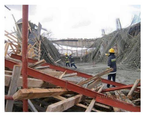
**Photo 8. 2:** The collapse of the roof of a building under construction during concrete pouring in Nablus<sup>109</sup>
