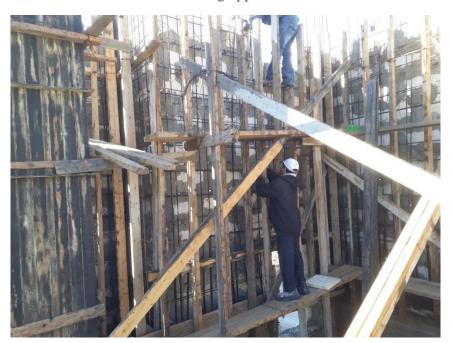
Photo 8. 5: Inadequate scaffolding system at a construction site in Ramallah
