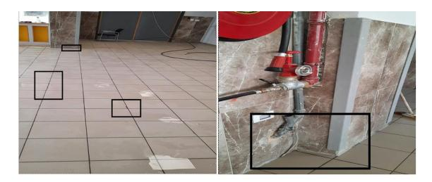
**Photo 9. 9:** the quality of floor and wall tiling in the project<sup>393</sup>
