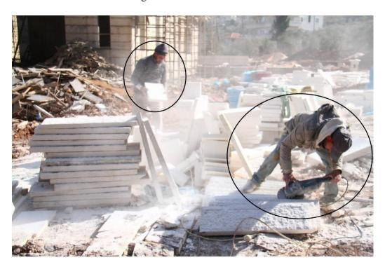
**Photo 9. 2:** Workers use an electric stone-cutter without any safety precautions
