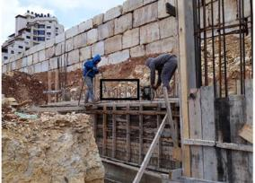
Photo 9. 4: Non-use of approved rebar safety caps during construction
