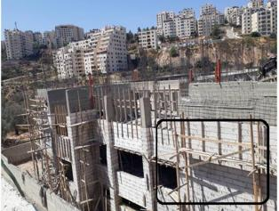
Photo 9. 5: Unsafe Tower scaffold used in the project
