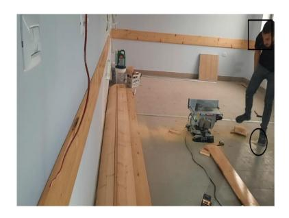
**Photo 9. 11**: A worker installing wooden cladding panels for walls<sup>396</sup>
