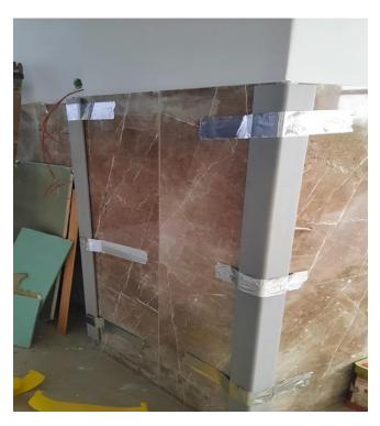
Photo 9. 10: Wall corner protection carried out by the contractor in the project<sup>394</sup>
