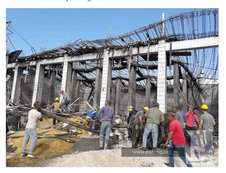
**Photo 8. 3**:The collapse of the roof of a building under construction during concrete pouring in Hebron<sup>110</sup>
