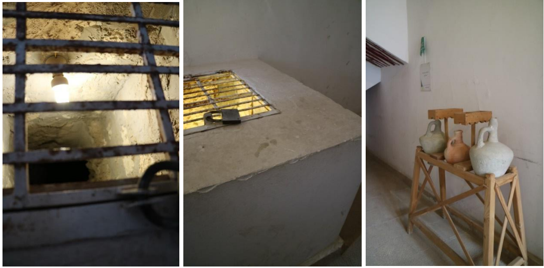
Figure 3.21: Water well located in the transitional corridor between the guest zone and the family zone (Source: Al-Jamea, 2016)
