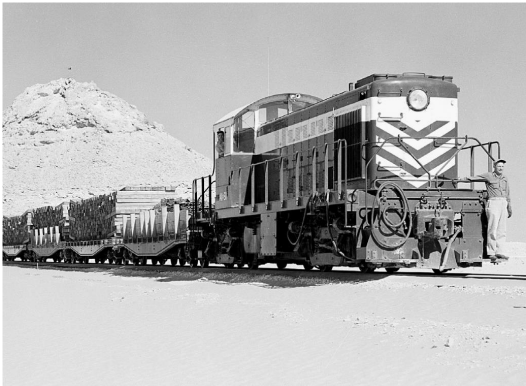
Figure 3.54: The newly established railway system transferring building (Source: Aramco, 2013a, p.13)
