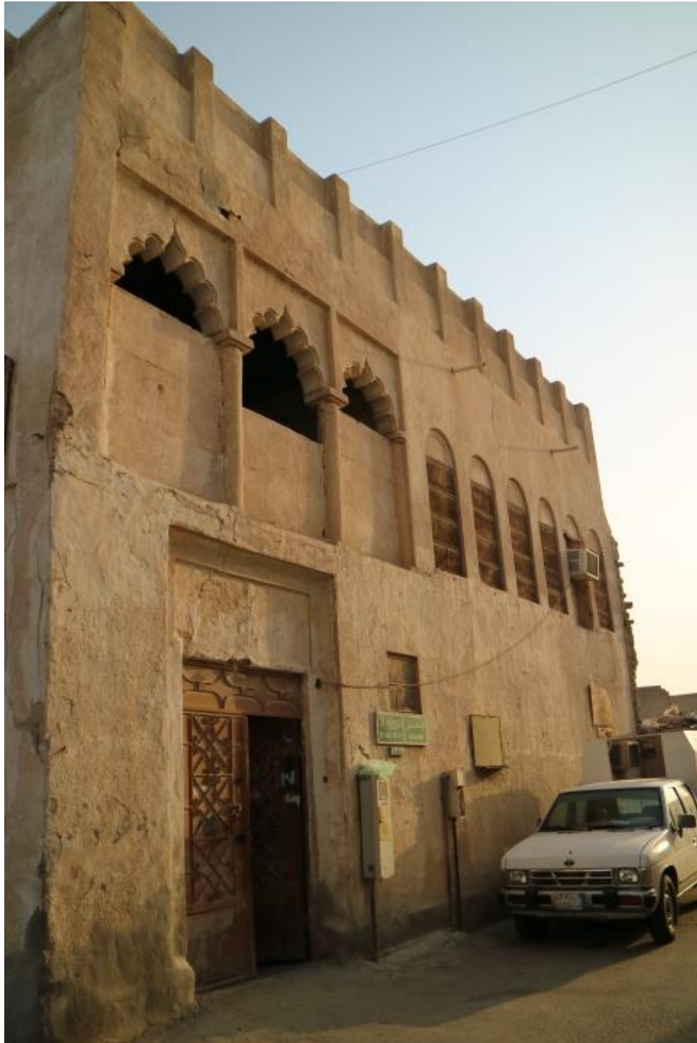
Figure 3.16: Rectangular façade form with arched windows
