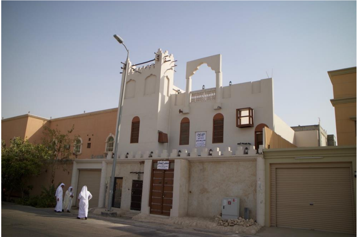
Fig. 6.48: Al-Naathil Museum's traditional façade existed in the middle of the contemporary villa's façade. (Source: May Al-Jamea, 2016)
