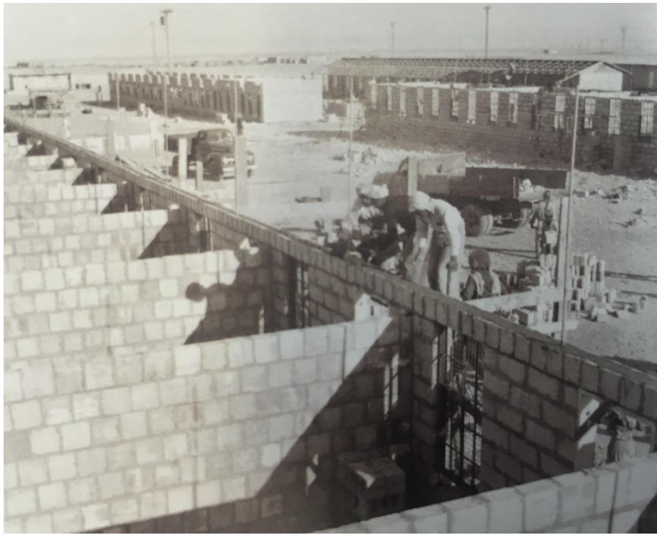
Fig. 3.52: Masonry construction was used for Saudi camp housing in Dhahran, 1952 (Source: Djaladin and Tahlawi, 1998, p.28)
