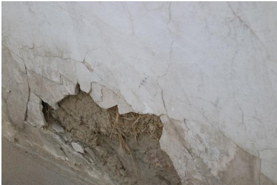
Figure 3.20: Mud construction appears in the lower part of the façade (Source: Al-Jamea, 2016)
