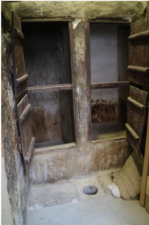
Figure 3.22: Date storage room and the open circular hole in the floor for the collection of date syrup (Source: Al-Jamea, 2016)
