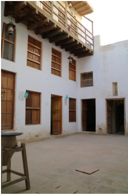
Fig. 6.44: Tiles on the floor of courtyard
