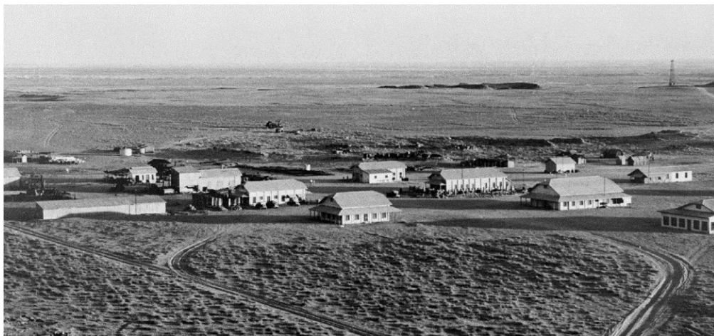
Figure 3.40: Dhahran oil camp in 1936 with a few buildings (Source: McMurray, 2011a, p.59).
