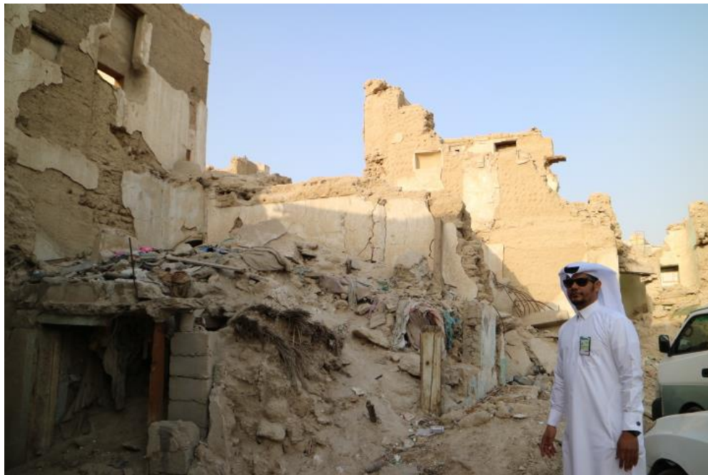
Figure 3.13: Remains of demolished Al-Naathil neighbourhood, reached with the assistance of Mr Al-Kuwaiti, a tour guide from the Saudi Commission for Tourism and National Heritage (Source: Al-Jamea, 2016)
