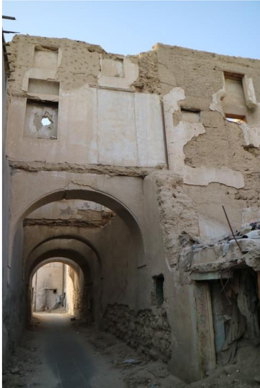
Figure 3.15: A sabat bridge area connecting two courtyard houses facing each other (Source: Al-Jamea, 2016)
