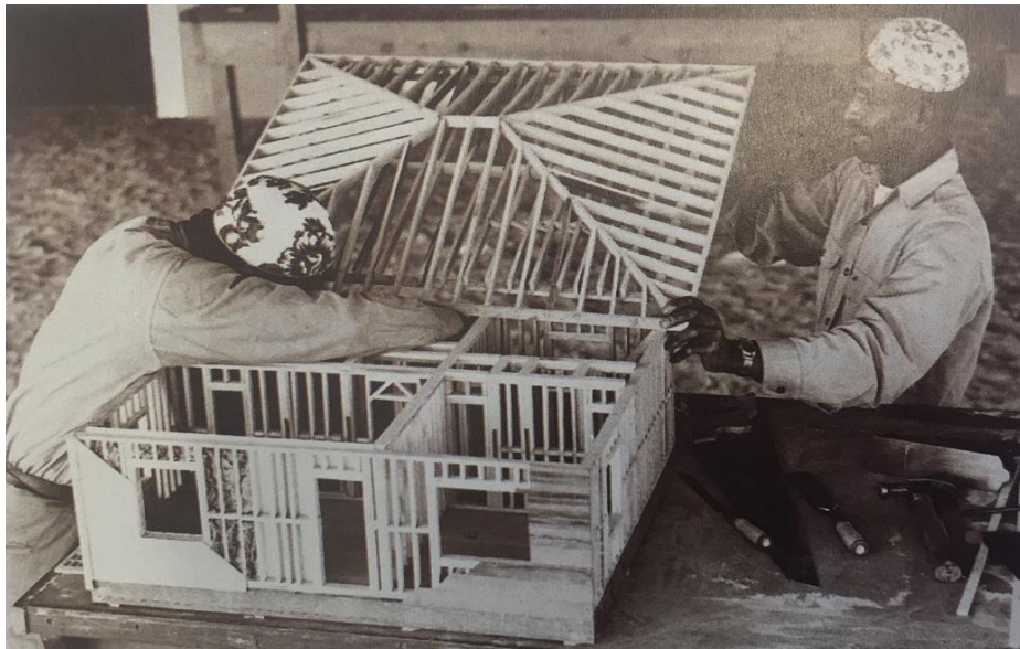
Figure 3.53: Working with a scale model to learn new construction techniques in 1950 (Source: Djaladin and Tahlawi, 1998, p.44)
