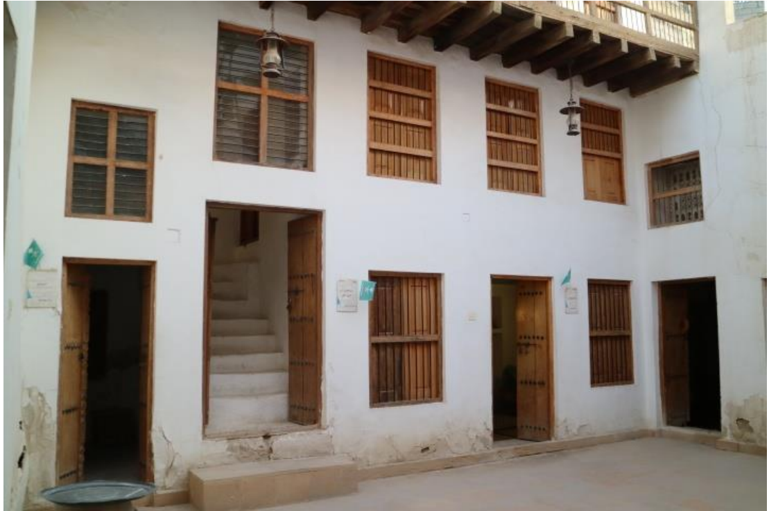
Figure 3.24: The family courtyard. All the bedroom doors and windows on the ground and first floor open onto the courtyard, with the far-left door leading to the kitchen (Source: Al-Jamea, 2016)
