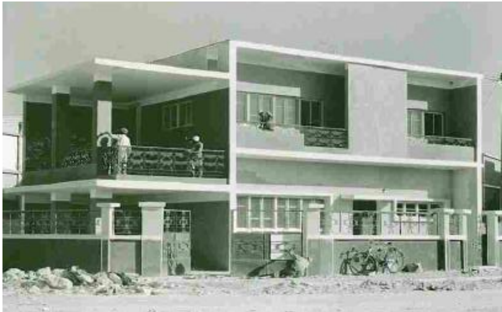
Figure 3.47: Finishing touches being put on a villa type house for an Aramco employee who had become the owner through the company Home Ownership Program in 1961 (Source: Pakka, 2006)
