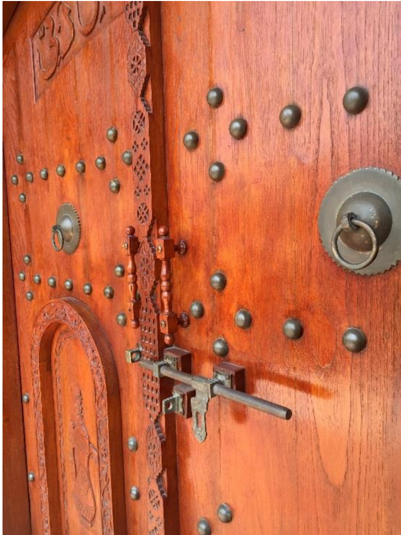
Fig. 5.21: The gate with two door knockers, a linear metal lock, decorated with a number of large metal studs. (Source: May Al-Jamea, 2014)
