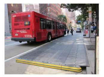
Figure 4.12: Temporary bus boarding platform in Pittsburgh, US. Image © Zicla.
