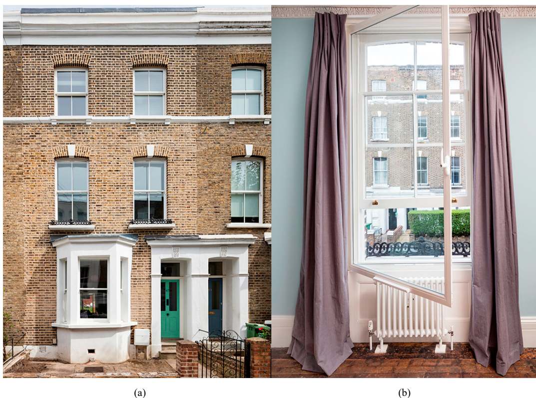
Fig. 1. (a) Front view of the property; (b) double glazed secondary window.
