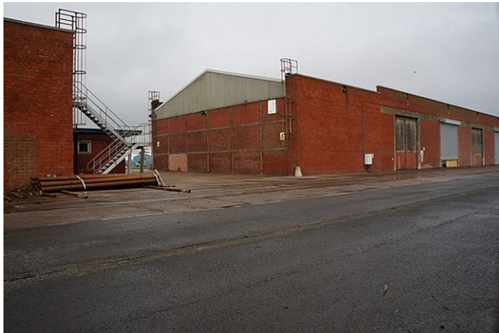
Post-war warehouse in dock area in Hull
