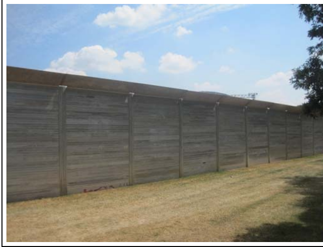
Figure 6. Super Fortress Fencing for the Lovebox festival in Gunnersbury Park in 2018. This is the most secure fencing available to festival organisers, and features tamper proof fitting and integrated gates. Super Fortress fences were developed by Eve Trakway, the industry's leading supplier of temporary fencing, and were first used at the Glastonbury Festival in 2002 as a response to the high volume of people breaching fences at the 2000 edition. Photo: Andrew Smith.
