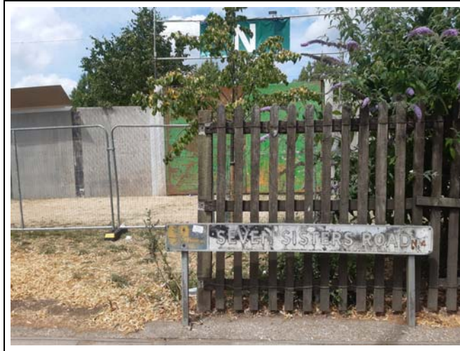
Figure 1. The multiple layers of fencing in Finsbury Park during the Wireless music festival in July 2022. Basic wooden fencing round the park is reinforced with a further layer of 2 m high anti-climb mesh panelling and the festival perimeter within the park is secured by 4.12 m high aluminium Super Fortress fencing. Photo: Andrew Smith.
