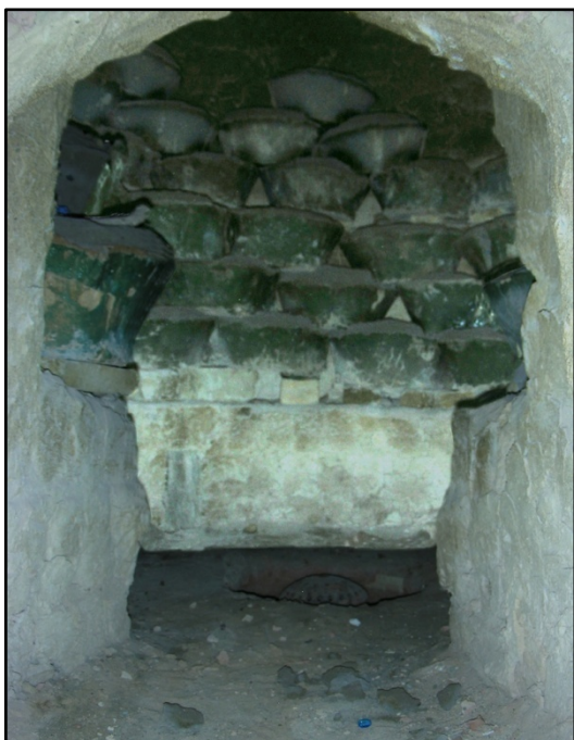
Figure 56: The kiln interior showing the stacked containers and the gas burner in the floor
