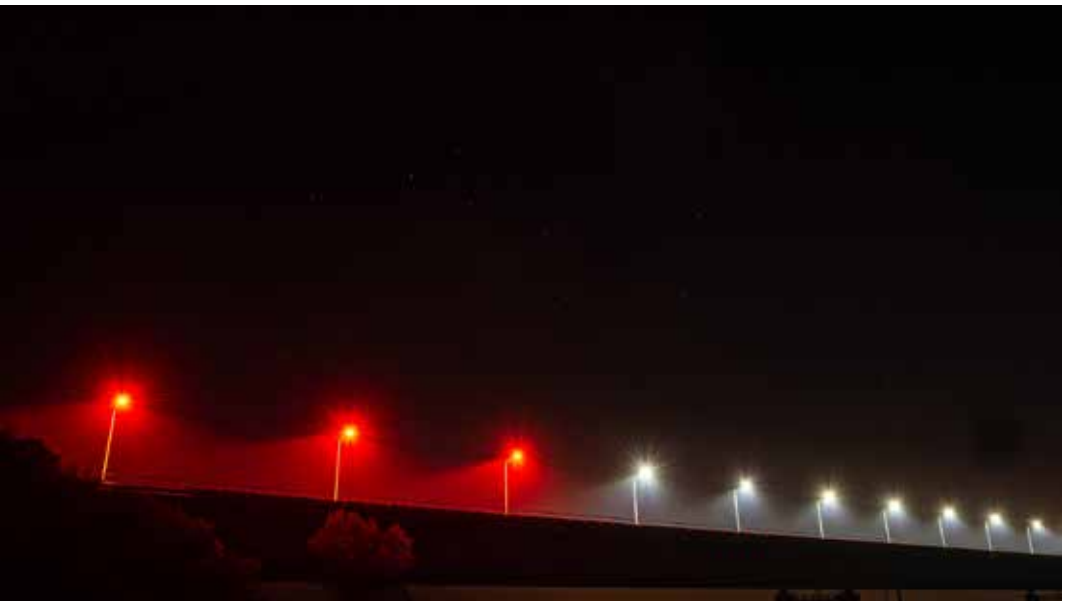
Figure 10 The red streetlights use a spectrum that is friendlier to both bats and moths. © Compass. https://www.compass.nl .
