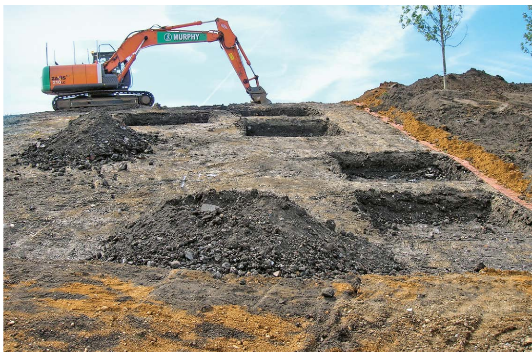
Figure 4 Tree pits being dug in the 'cleansed' fill prior to the marker layer and imported soil being installed. The full profile is visible to the right of the image.
