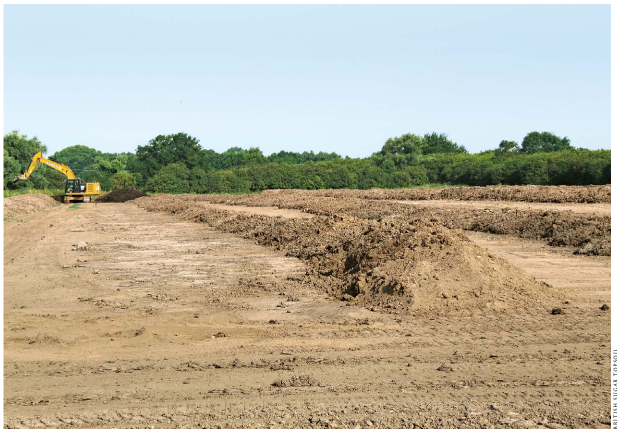
Figure 8 Soil drying process, 2020.
