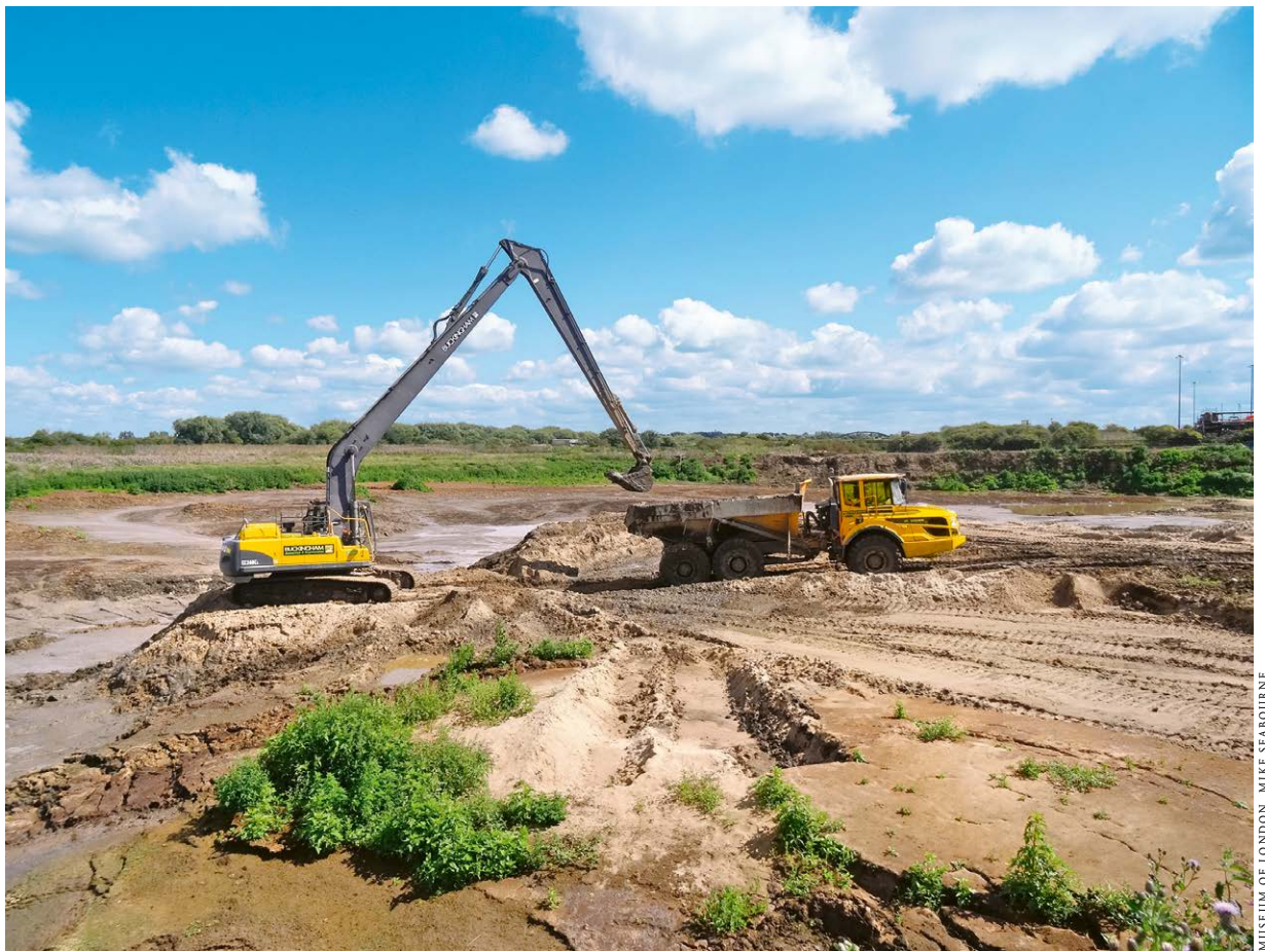
Figure 6 Settlement lagoons being emptied at British Sugar Topsoil's Wissington site, 2020.
